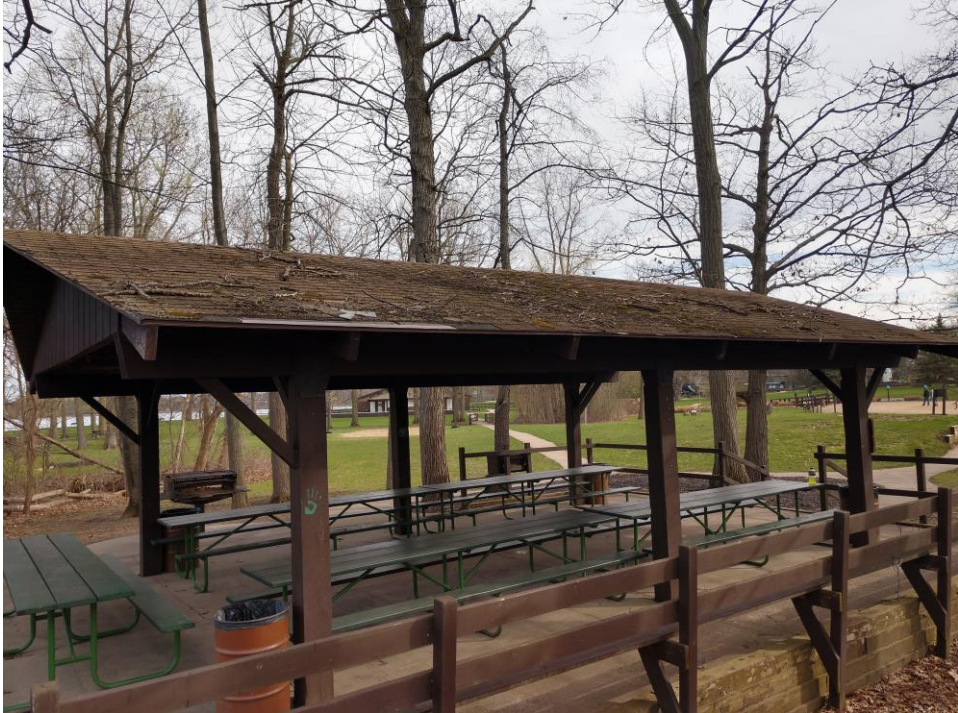
LAKE LANSING PARK - SOUTH (LAKEVIEW PICNIC SHELTER)
